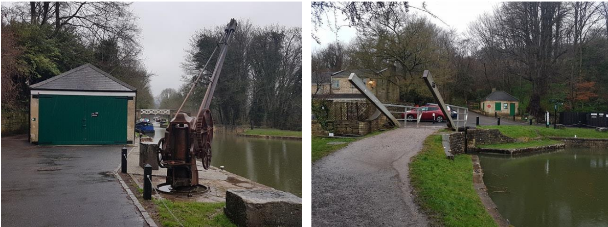
Figure 11: Dundas basin – interpretation of old canal structures at the towpath entrance to the Somerset Coal Canal
